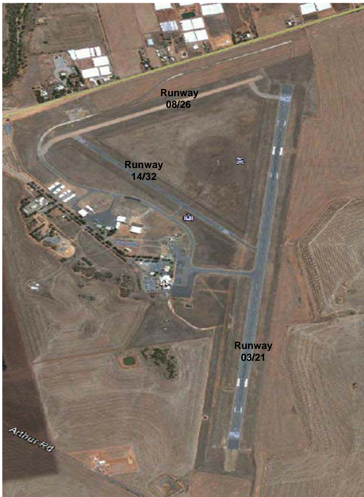
Geraldton Airport Runway Infrastructure
